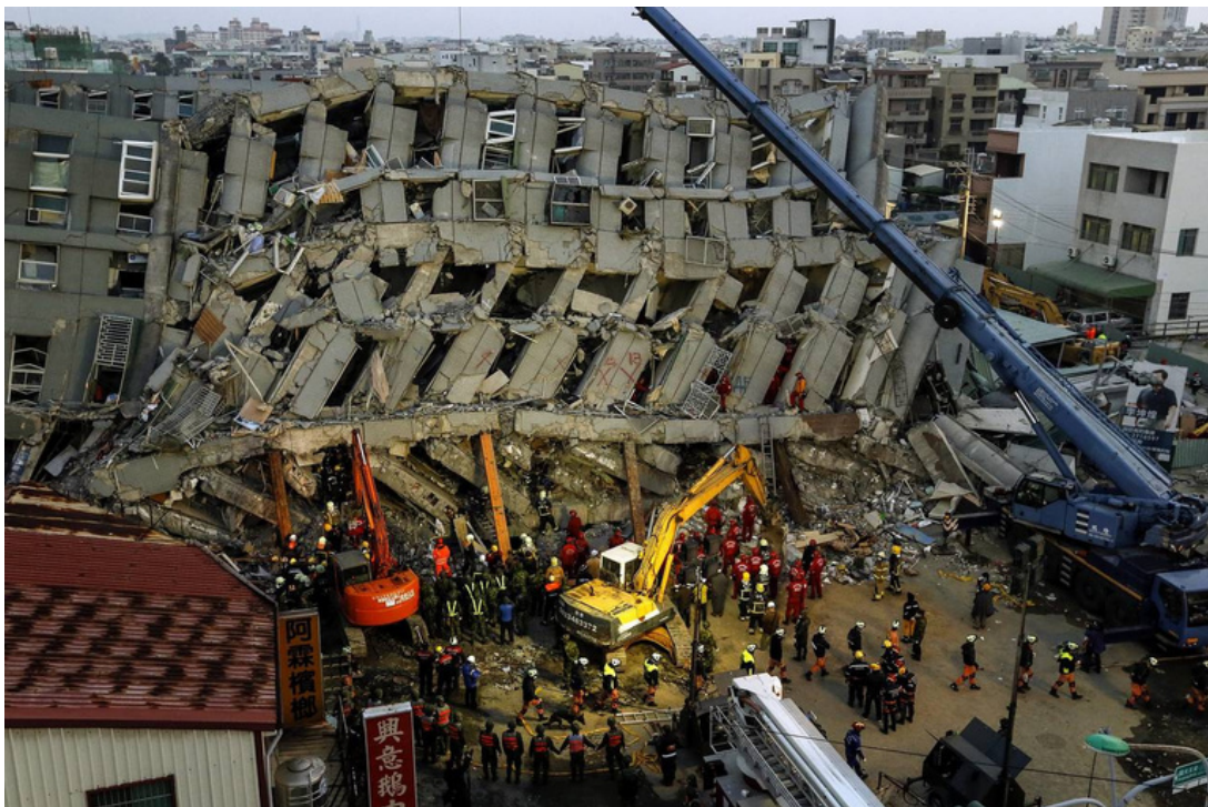
Collapsed building during the 06.02.2016 earthquake in Taiwan, Mw 6.4 Source: https://www.wsj.com/articles/taiwan-officials-launch-rescues-1454816862
